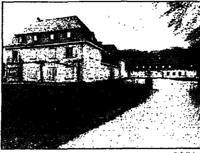
The Chateau de Betzdorf before the start of renovation.
